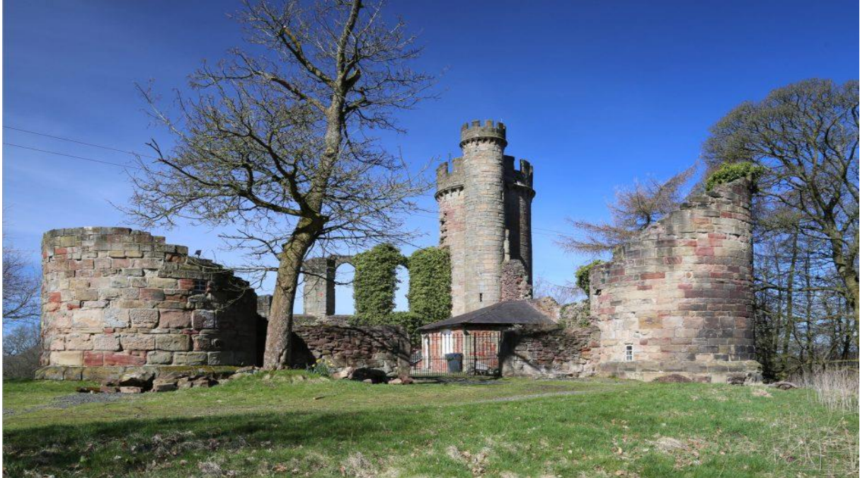
Şekil 6. Sanderson Miller, Hagley Castle , 1747/48, Hagley Park, Worcestershire.
